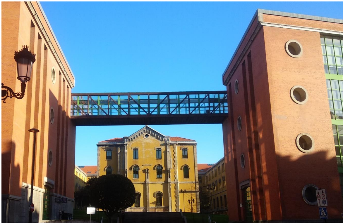
Figure 1. Pedestrian Footbridge at the Milan’s campus.
