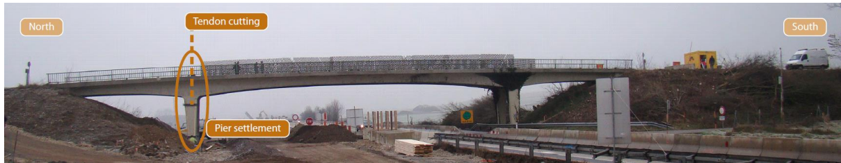
Figure 8. The S101 bridge. Locations of introduced damage are marked in the figure around the north side pier ( www.vce.at/iris/ )
