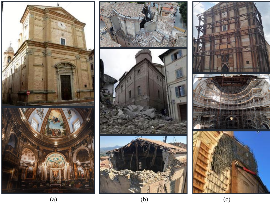
Figure 1. The Santa Maria in Via church: (a) pictures before the 2016 earthquakes; (b) damage suffered after the seismic sequence, (c) securing systems.
