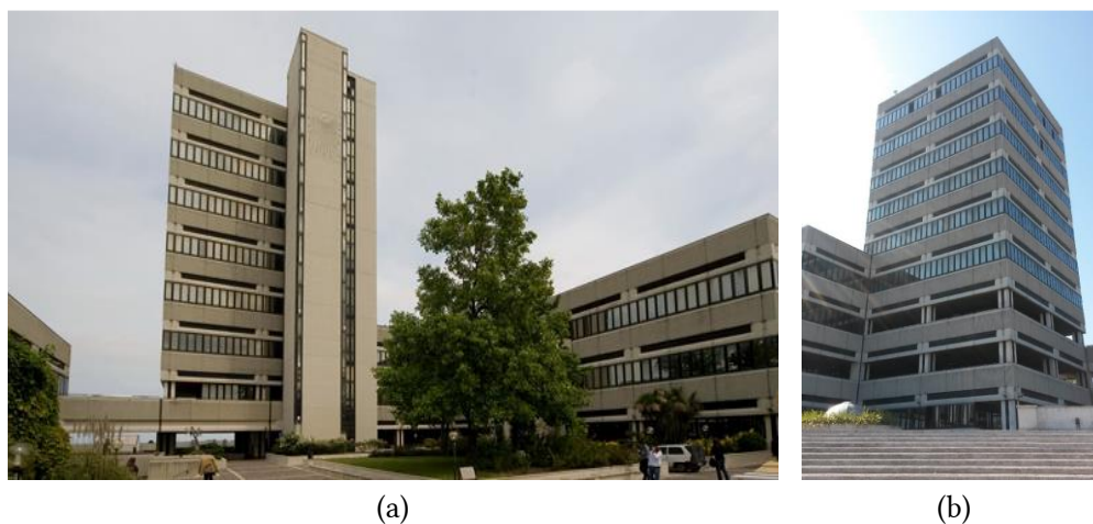
Figure 1. View of the tower: b) South c) and North-West views.
