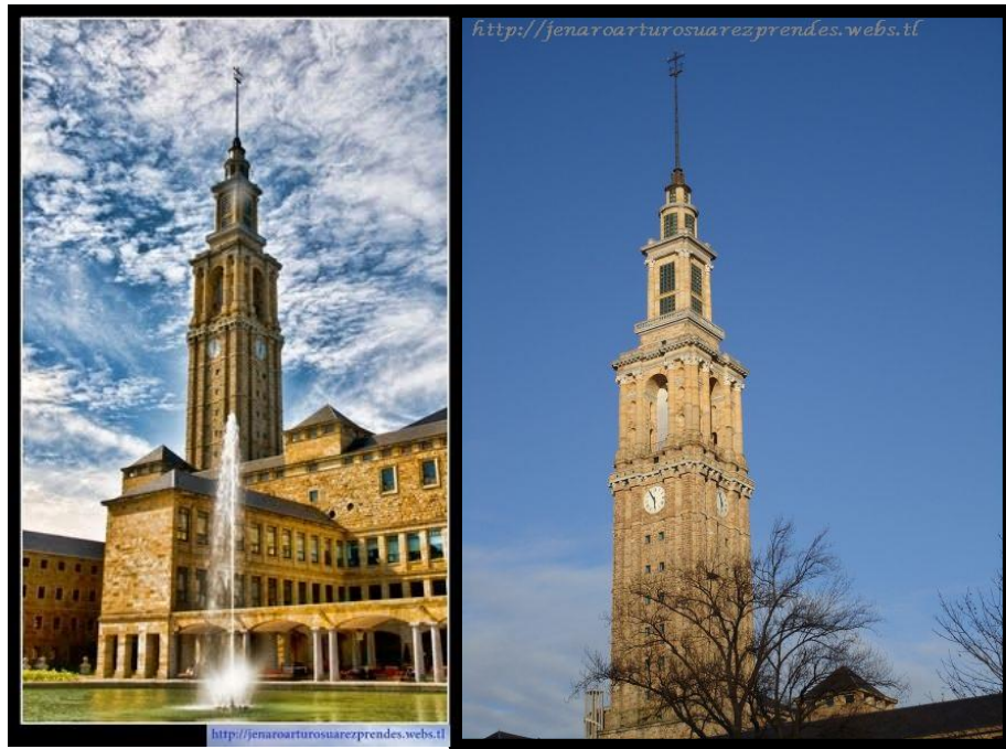
Figure 2. Views of the Tower (from https://jenaroartirusuarezprendes.webs.tl )
