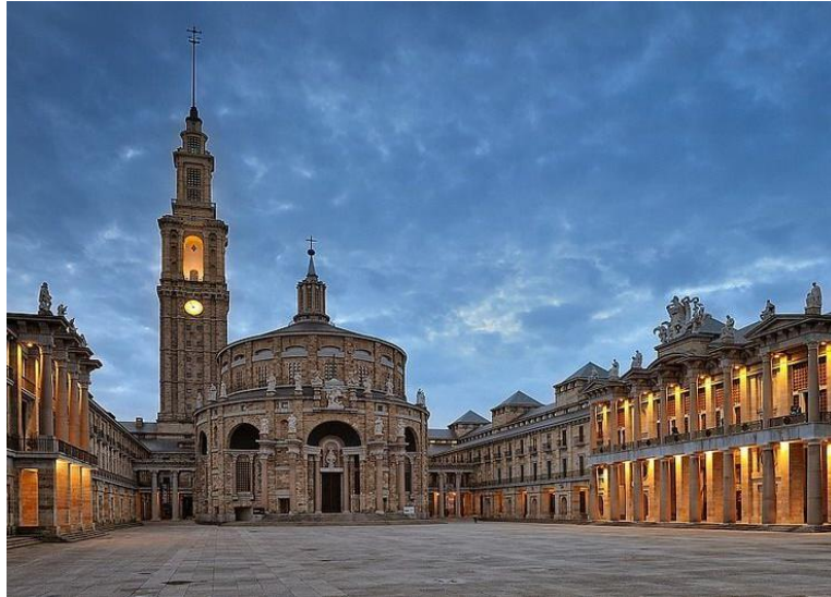
Figure 1. “Laboral City of Culture” Building (Gijón-Spain)
