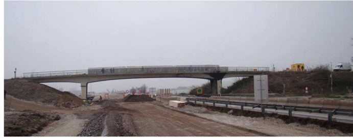
Figure 1: S101 Bridge before demolition.
